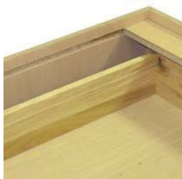
Particleboard Construction (back detail)
